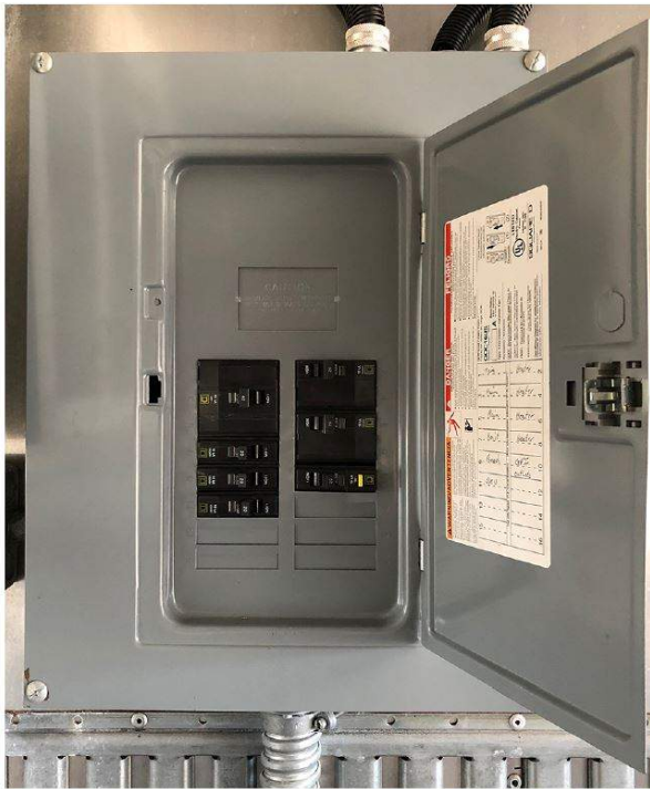
Figure 1-12. M-van power distribution panel.
