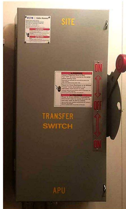
Figure 1-4. PMT van power transfer switch.
