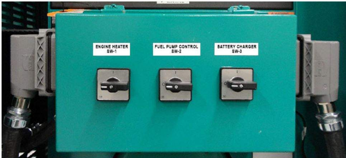
Figure 1-15. Wing 1 LF DEU interface panel.
