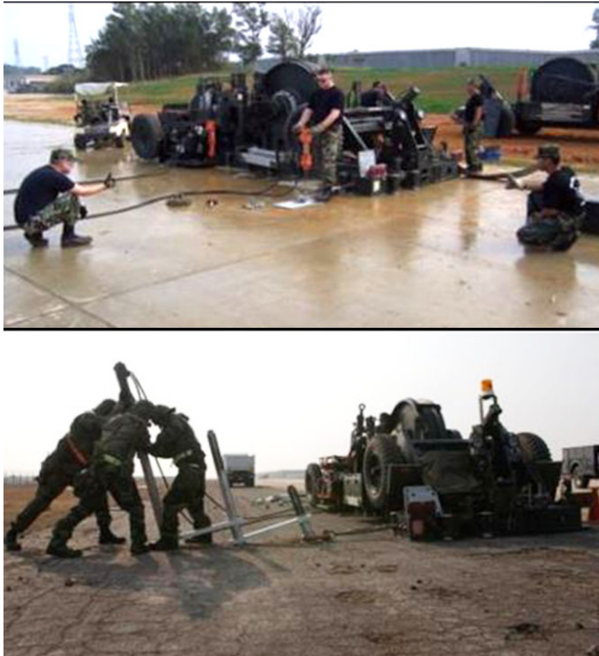
Figure 2-62. Concrete MAAS install (top) and soil install (bottom).
