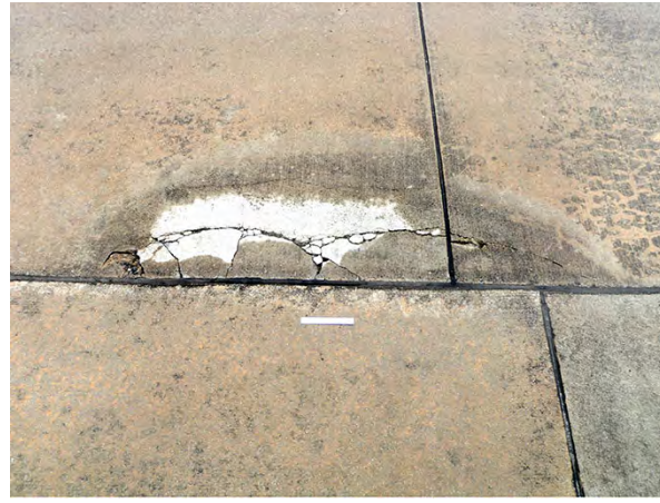
Figure 3-10. Spalling.
