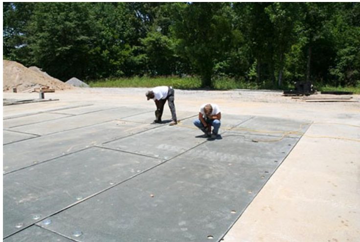
Figure 2-4. Assemble FRP mats.
