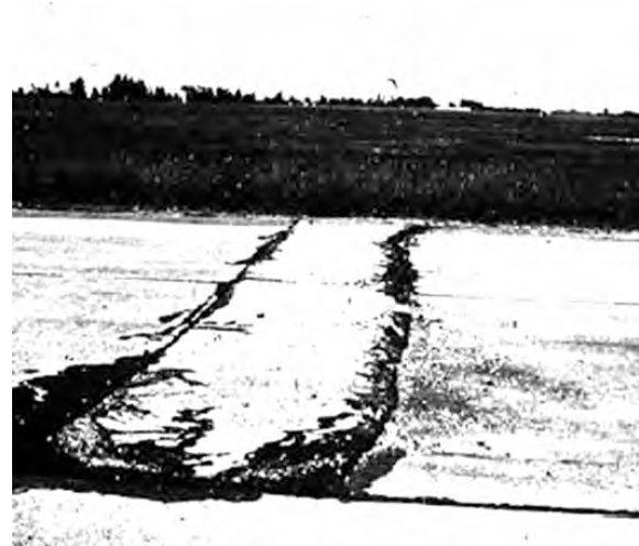
Figure 3-14. Concrete blowup.
