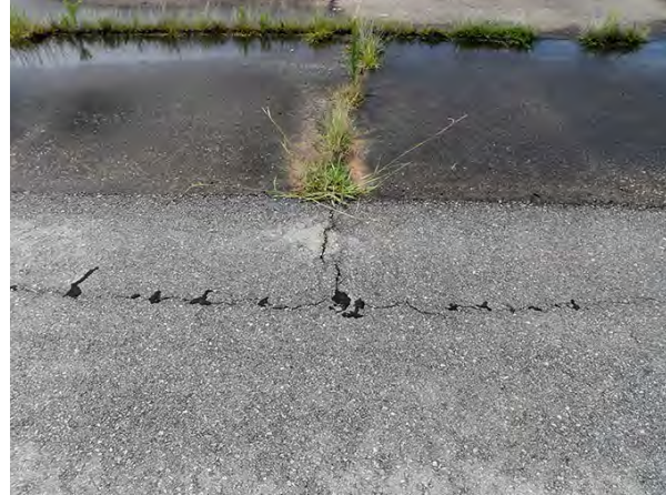
Figure 5–2. Edge cracks.
