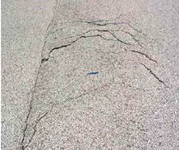
Figure 5-7. Slippage cracks.
