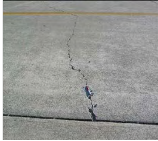
Figure 3-4. Transverse cracking.
