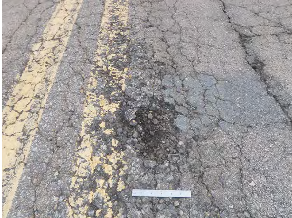
Figure 5–1. Alligator cracks.
