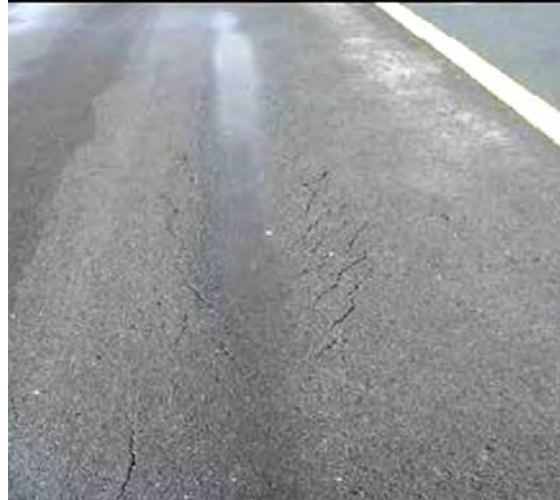
Figure 5-8. Channeling or rutting.
