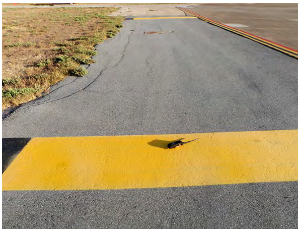
Figure 5–3. Edge-joint cracks.
