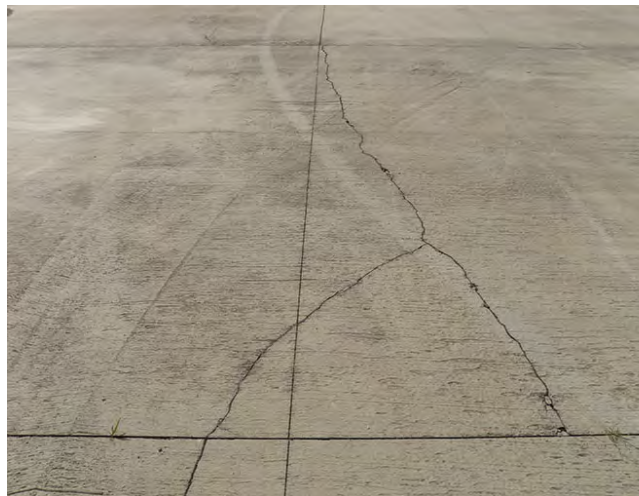
Figure 3-6. Diagonal crack.
