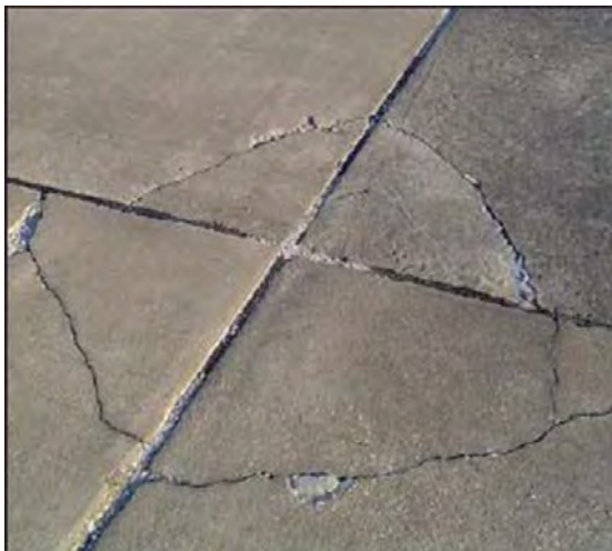
Figure 3-5. Corner crack.
