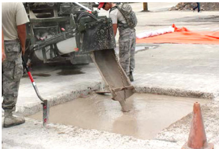
Figure 1-27. Backfill under asphalt cap nearing completion.
