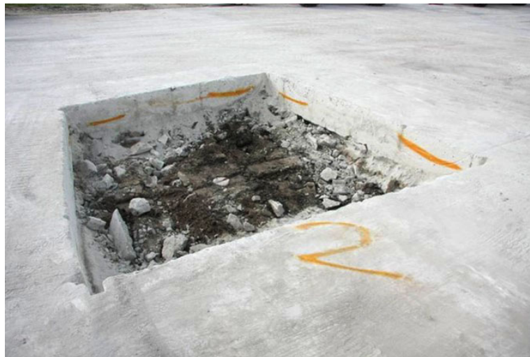
Figure 2-3. Remove damaged pavement.
