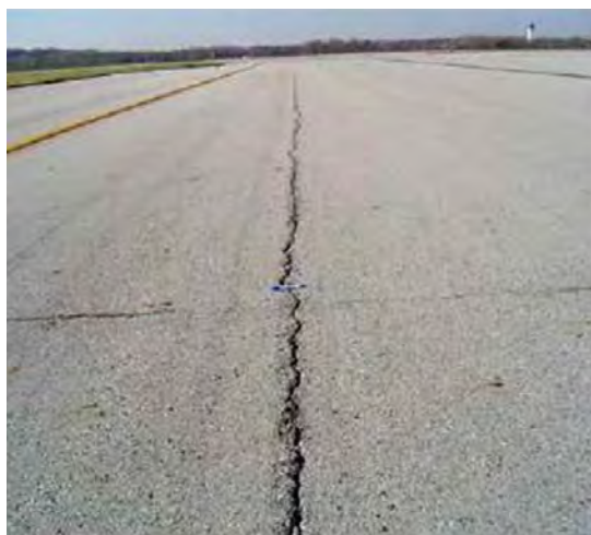
Figure 5-5. Reflection cracks.
