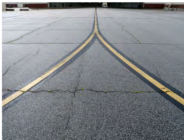
Figure 5-6. Shrinkage cracks.
