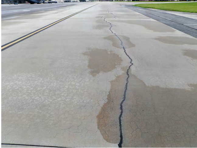
Figure 3-3. Longitudinal cracking.
