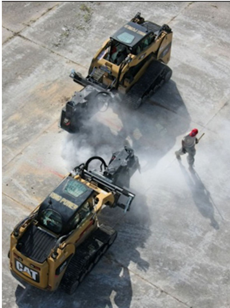
Figure 1-15. Cutting parallel lines simultaneously.
