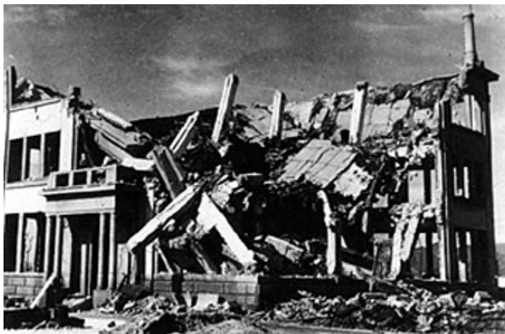
Figure 4-11. Blast effects on a concrete building at Hiroshima.
