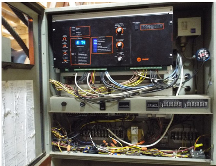
Figure 3-29. Chiller control board.
