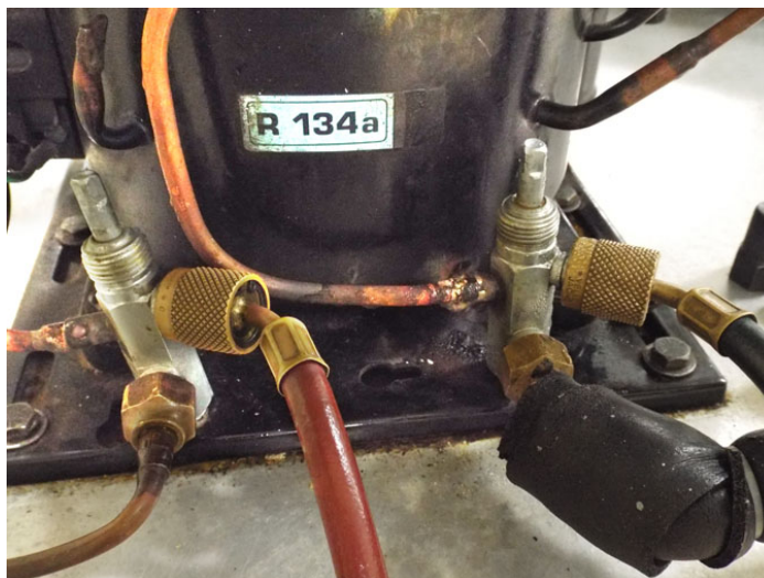
Figure 2-20. Service valves.
