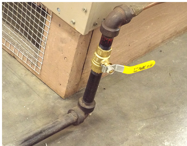
Figure 1–7. Manual shut off ball-valve.
