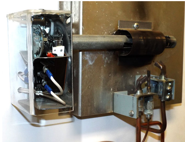
Figure 3-18. Combination fan-limit control.
