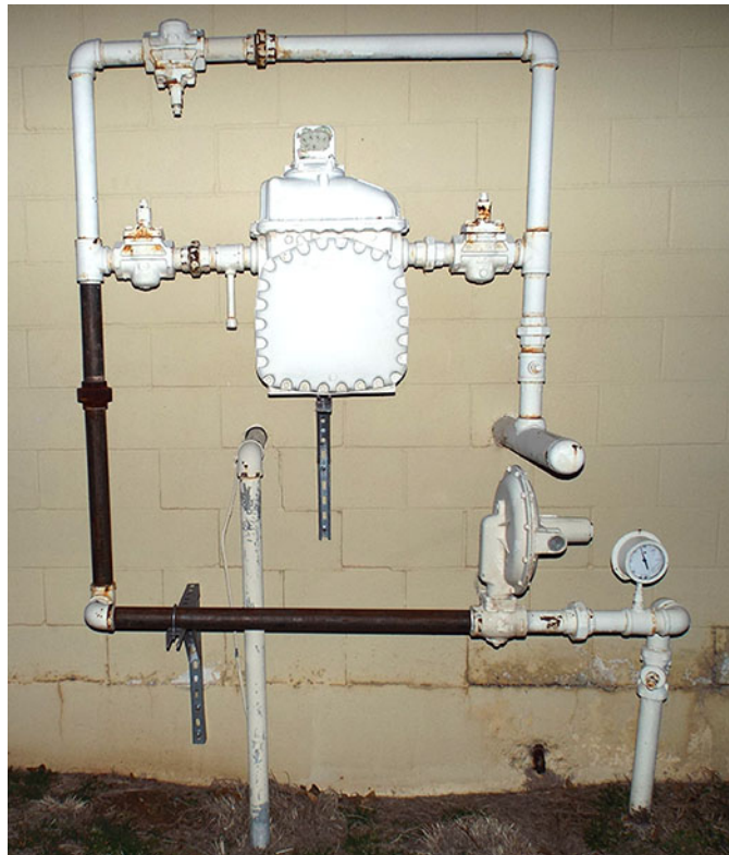
Figure 1-21. Building regulator.
