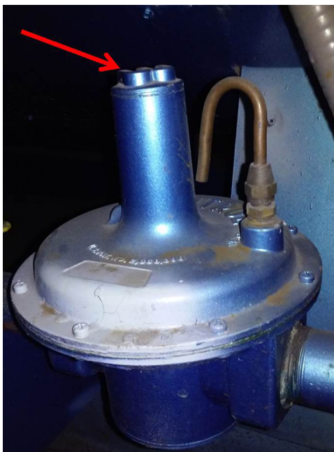
Figure 2-48. Regulator plug.
