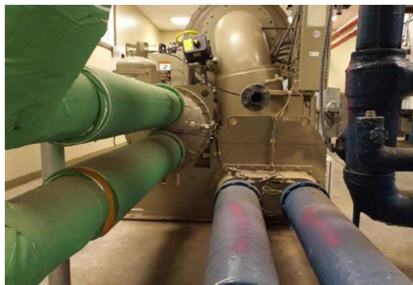
Figure 1–27. Shell-and-tube water-cooled condenser inlet and outlet front view.
