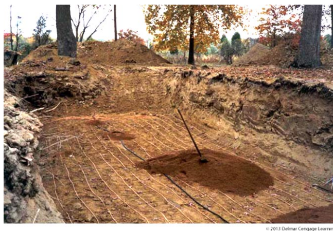
Figure 3-43. Diagonal drilling feeding pipe. (Courtesy Earthlinked Technologies.)
