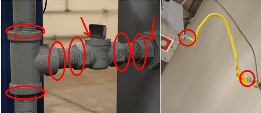
Figure 1-23. Gas line fittings to check.
