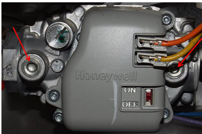
Figure 2-50. Gas ports.
