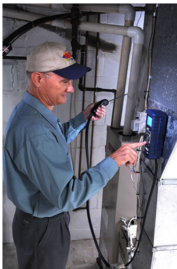
Figure 2-10. Checking flue gas temperature/efficiency on gas installation. (Reprinted by permission.)
