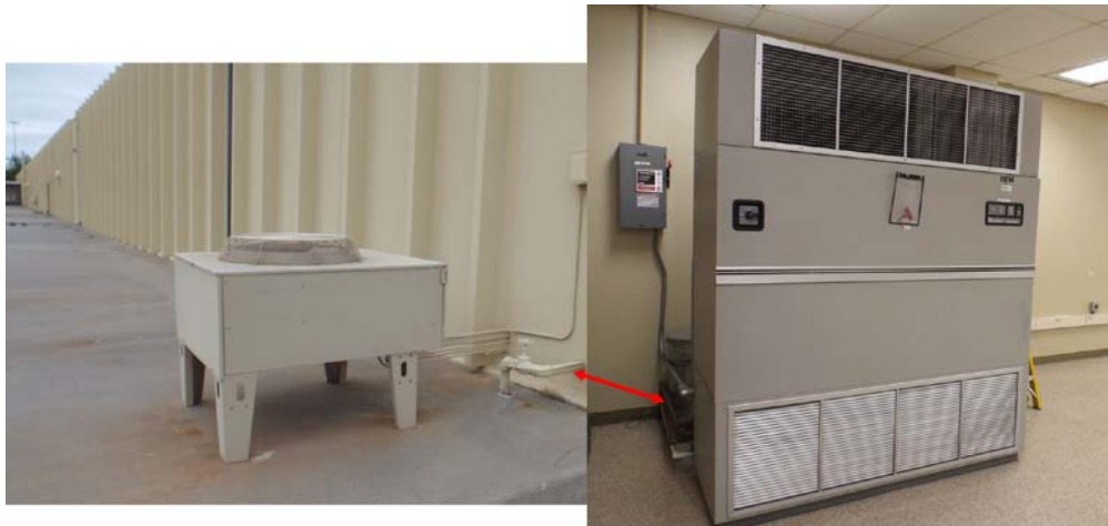
Figure 3-8. Outside and inside unit of split system.
