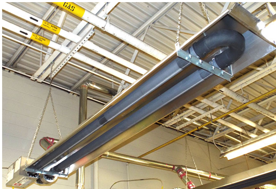
Figure 3-21. Radiant tube heater.
