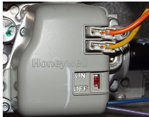
Figure 2-17. Gas valve wires from control board.
