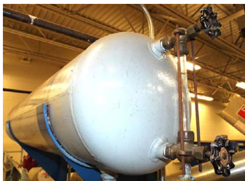
Figure 4-37. Expansion Tank.
