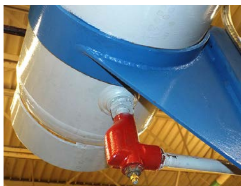
Figure 4-36. Air vent valve.
