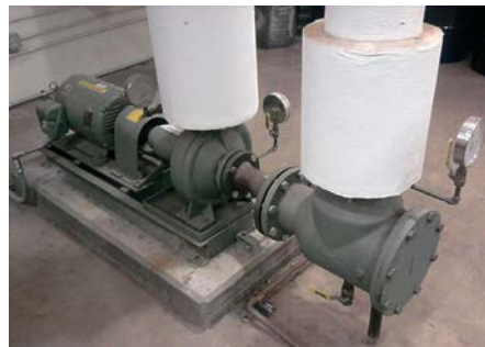
Figure 3–32. Chilled water pump.
