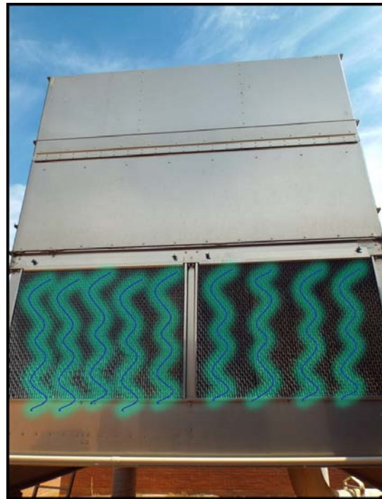
Figure 1-33. Fill material water trickling.
