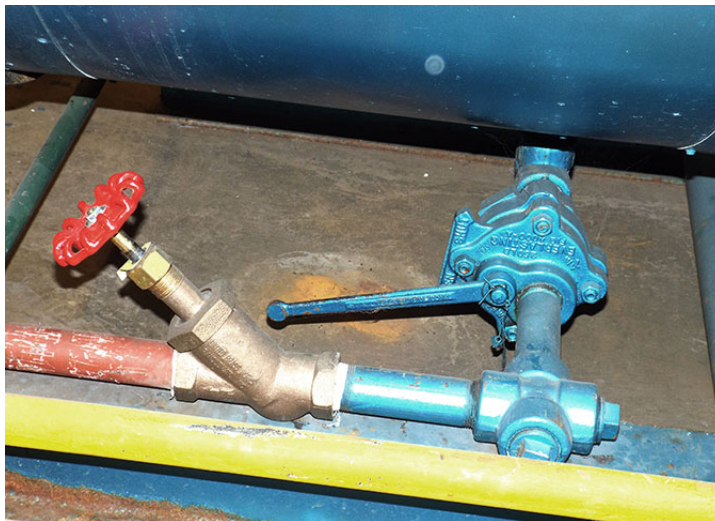
Figure 4-8. Tandem blowdown valve.
