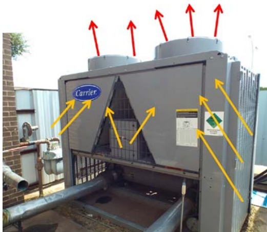
Figure 1-20. Air-cooled condenser air flow on a chiller.
