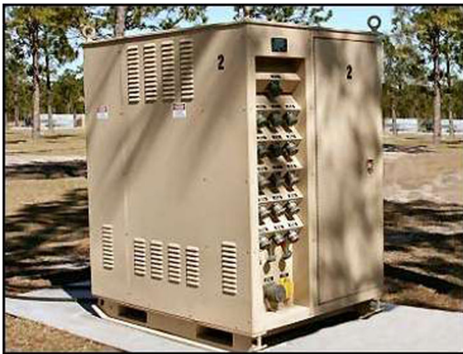
Figure 2-3. Primary distribution center.
