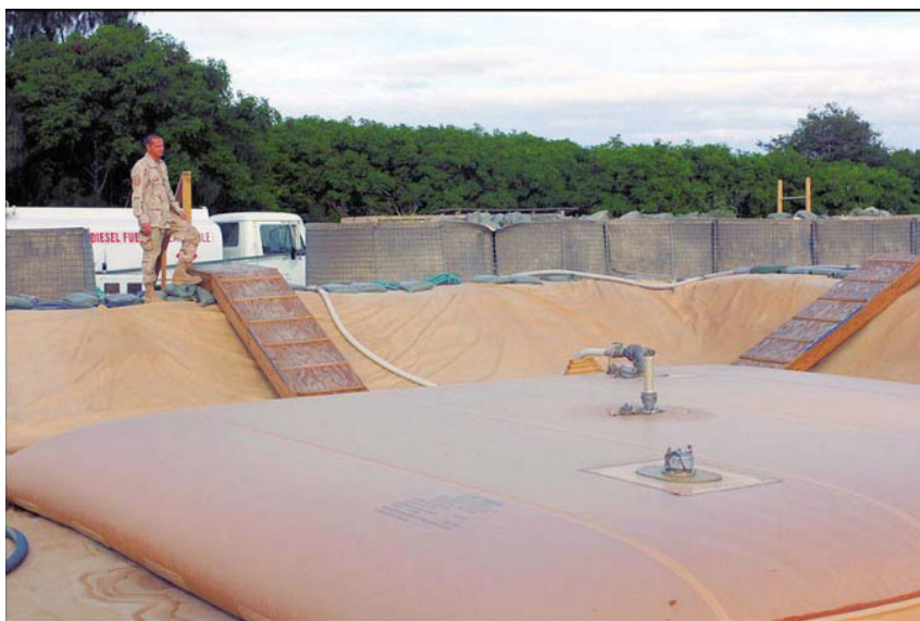
Figure 1-5. Power plant fuel bladders.
