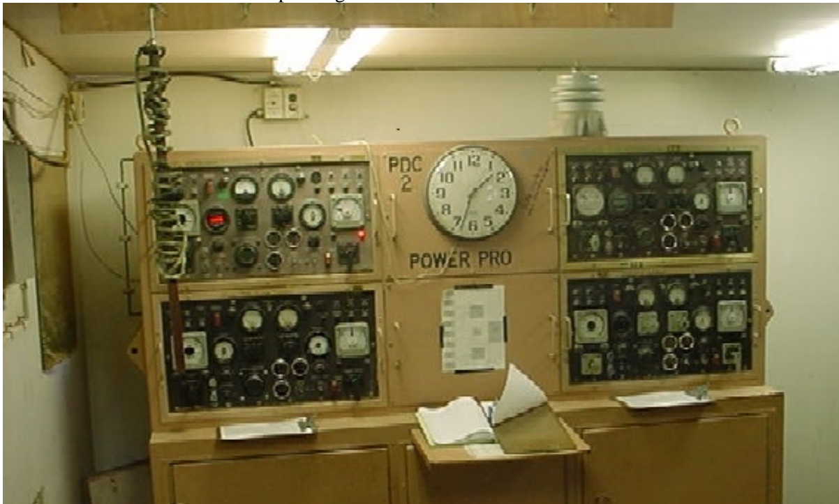
Figure 1-26. MEP-12 control rack.
