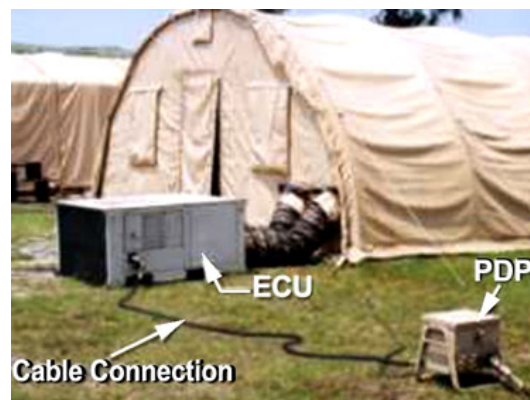
Figure 2-12. Secondary power cable connections to ECU.
