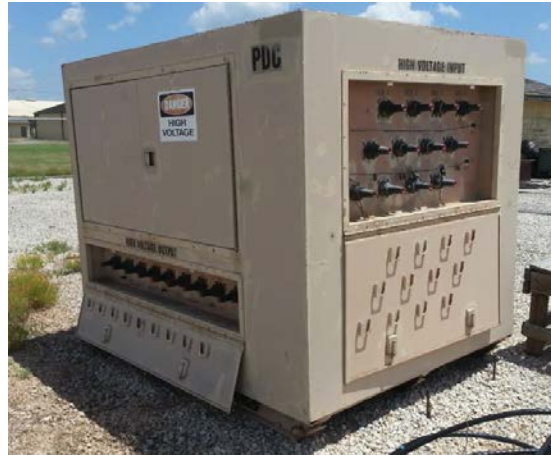
Figure 1-11. Primary distribution center.
