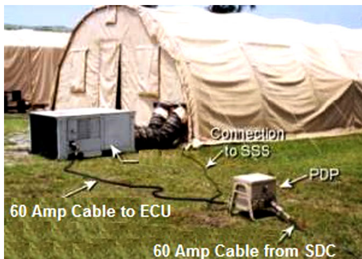
Figure 4-39. Secondary cable connections.
