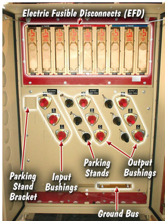
Figure 4-31. SDC high voltage compartment.
