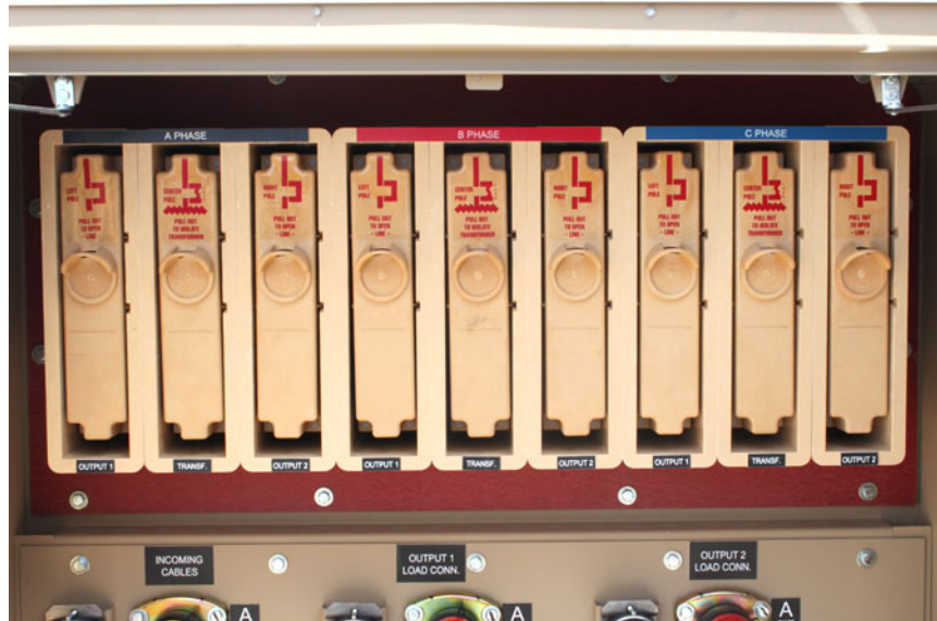
Figure 4-32. SDC high voltage compartment.
