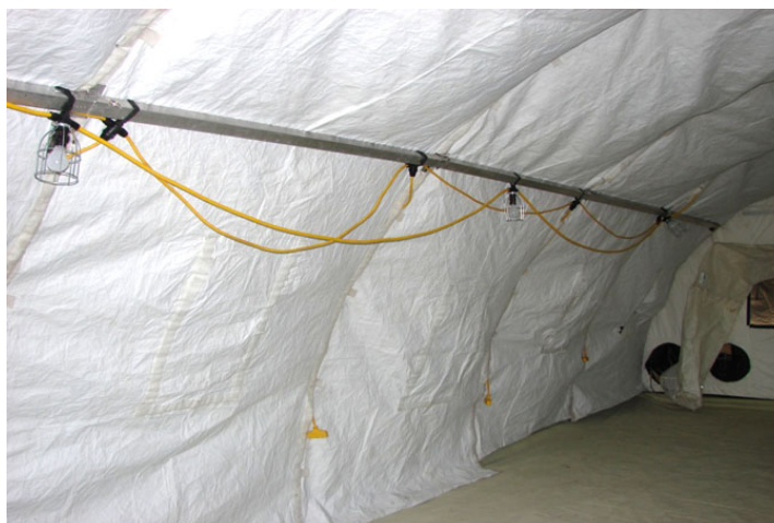
Figure 4-47. Lighting streamer.
