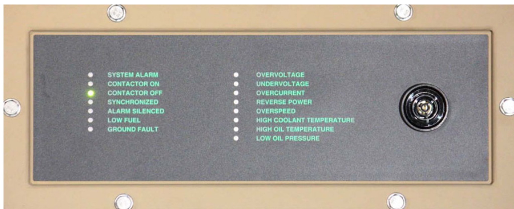
Figure 4-4a. Fault annunciator.
