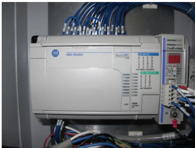
Figure 3-17. ROWPU PLC.
