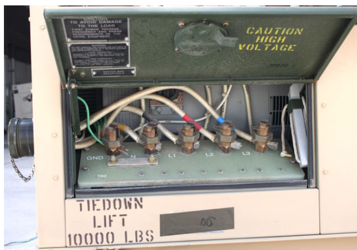
Figure 2-5. Generator connections.
