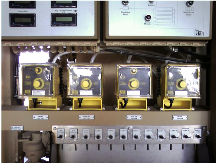
Figure 3-23. ROWPU chemical feed pumps.
