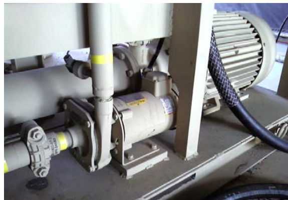
Figure 3-20. RO and Booster water pumps.
