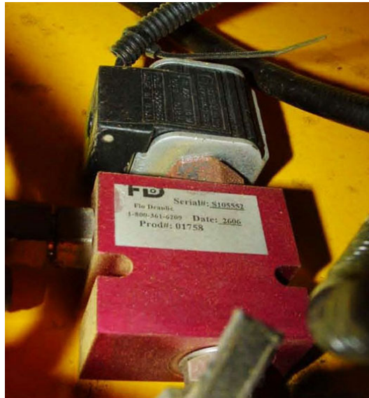
Figure 1-22. Pilot cut-out solenoid valve.
