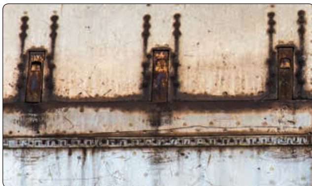
Figure 8-18. Galvanic corrosion.
